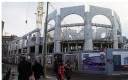
The Dutch Way'. Plattenbau over everything. The only JOA robot columns, in 23 years, that were useless for servicing from the interior! They were filled with pre-cast concrete! Ironically, it was this pre-cast, which no-one sees, that prevented the early erection of the JOA Entablature of blue logs, black caps, etc.. No Entablature = No Roof. No Roof = No Interior for six months. A failure of the builderly imagination - by the Project Manager.
