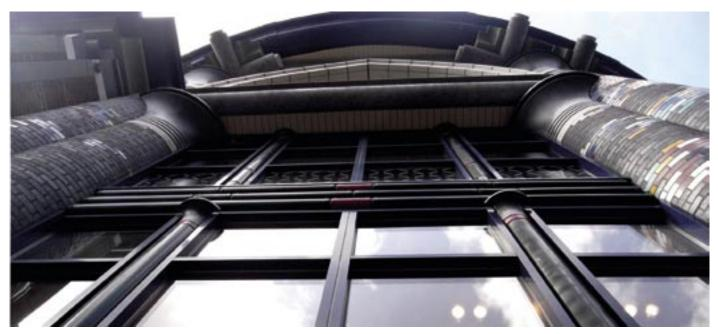
The previous picture, and this one, shows the big white arches.. Marbra-Lys cast the arches in two halves, with their faces laid flat on the floor. They come to a feeble point, when seen in 3-D, rather than a proper half-circle. The contract drawings showed the arch to be 'curved-on-curved work, rounded on plan. Again Marbra-Lys cheated, the Dutch Architects, INBO, ignored the fault and MAB did nothing. JOA were not even allowed to inspect the castings.
